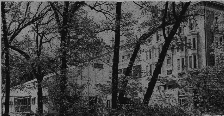
THE COURT WHERE BADGER coeds have played tennis in the shadow of Chadbourne Hall for 75 years is now the site of an ex-Army building which will be used as an emergency laboratory. The temporary structure is one of 26 now scattered over the campus.
