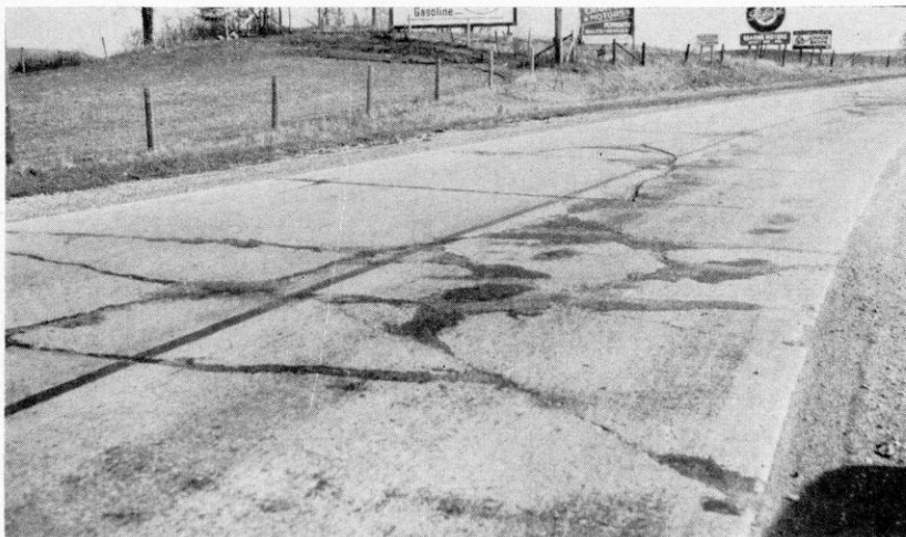
Figure 11. Highway pavement over Clyman silt loam, a naturally somewhat poorly drained soil with a seepage condition, which gives imperfect support to the highway. The pavement is in poor condition. (See units Nos. 4 and 18 on the colored soil map.)
