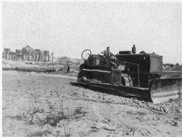
Blitzed areas were levelled with imported American bull-dozers to help West Berliners plant small vegetable gardens and beat the attempted Soviet starvation blockade.
