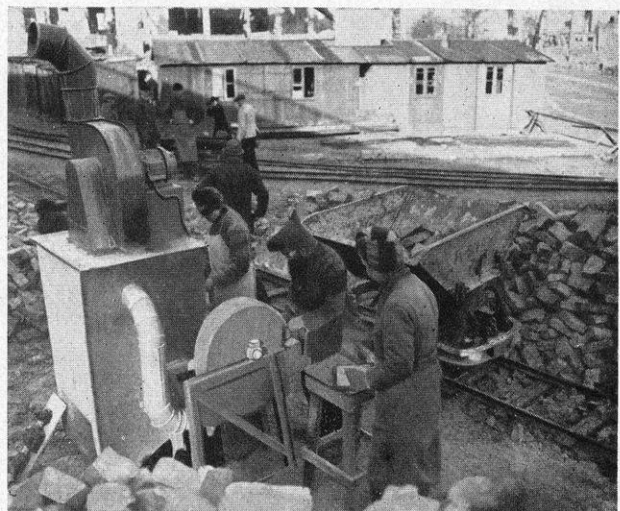
Bricks, which once made up the walls of a million Berlin homes, are processed to make well-surfaced new bricks—to build the walls of new Berlin homes.
