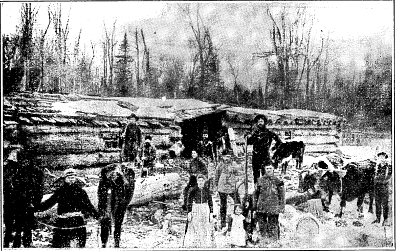
Note both the "shake" and "scoop" roofs of this Wisconsin logging camp.
