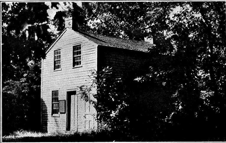
Built in 1842, "Blue House" at Nashotah was the first school of higher learning in Wisconsin. It is still standing.
