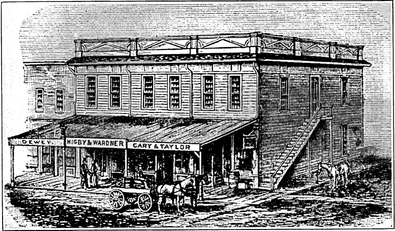
The Sentinel Building, Milwaukee, 1843.
