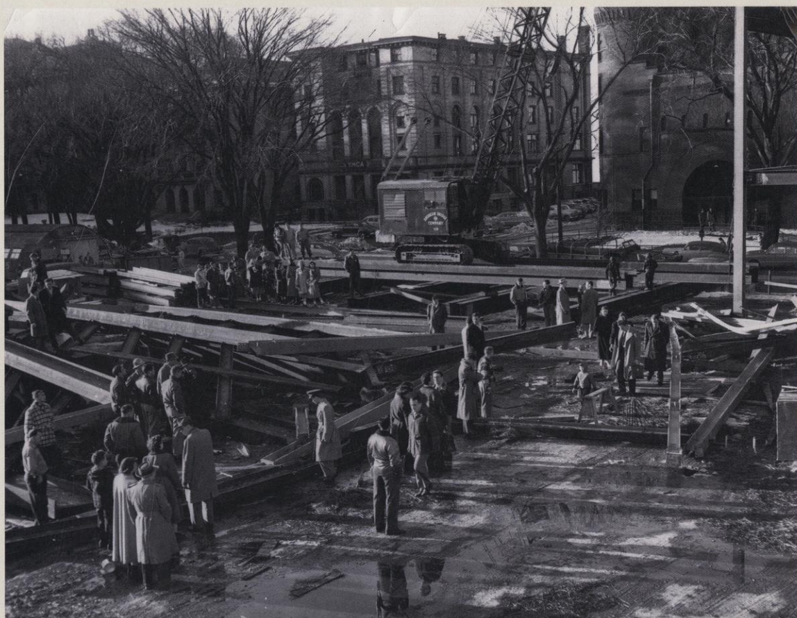
Right. This photo looking northwest across the first floor of Memorial Library was taken moments after the steel support structure collapsed the afternoon of March 16, 1951.
