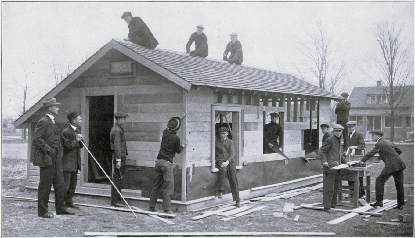
PROBLEM IN CARPENTRY CONSTRUCTION BY HIGH SCHOOL MANUAL TRAINING CLASSES
