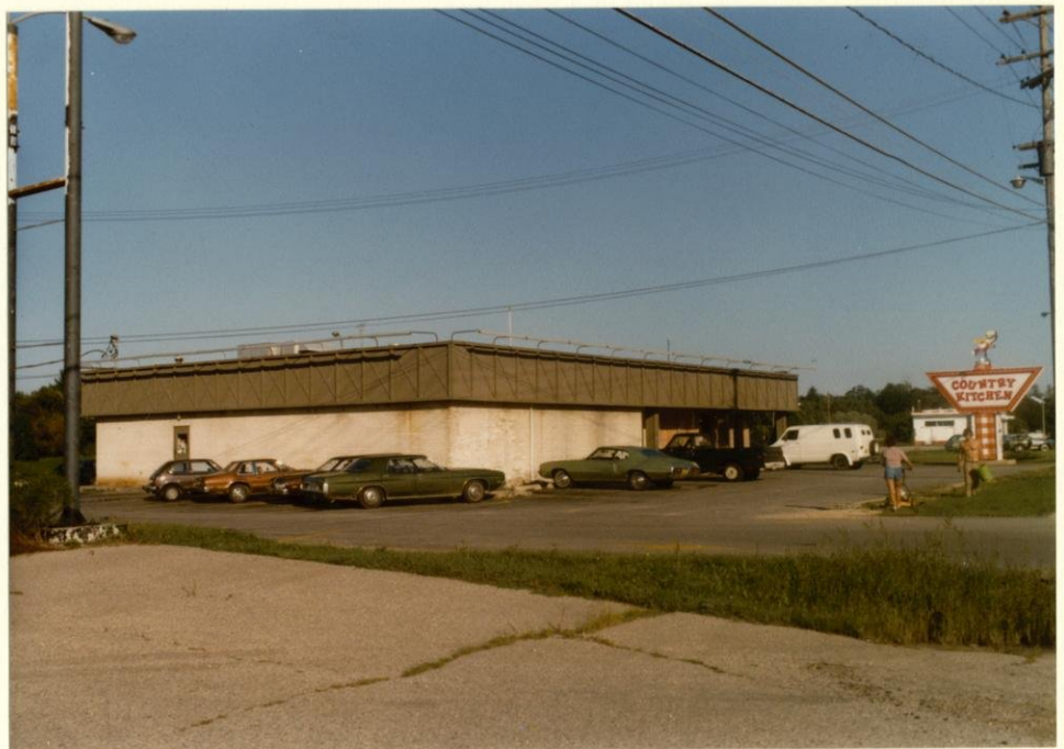
Taken from vacated Consolidated Station site looking east toward subject. South side of structure parallels University Ave.
