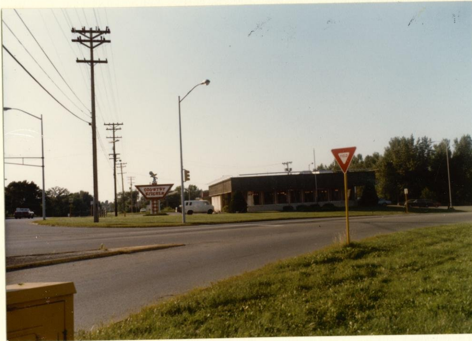
Looking west northwest from Allen Blvd. and University Ave. intersection. Proposed changes on Allen Blvd. include new right turn lane onto University Ave. which cuts through grassy strip in front of structure.
