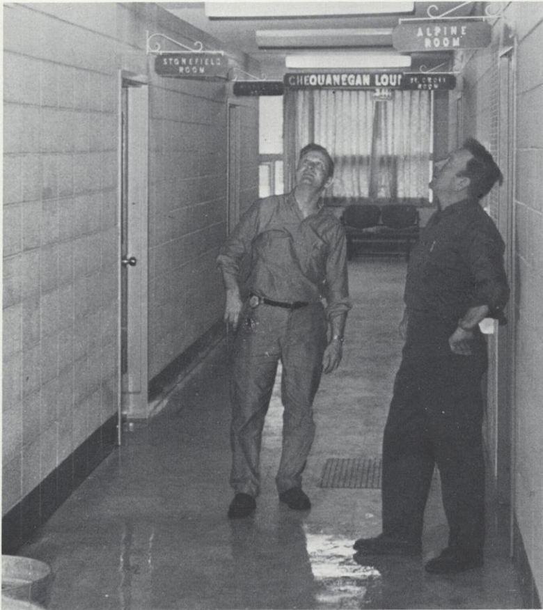
Janitors fixing the ceiling.
