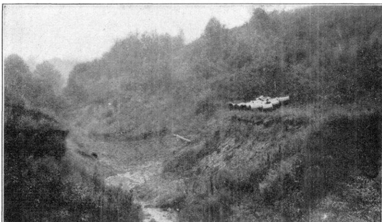
Fig. 5. Upper side of dam in gulley just made to cause filling of gulley. The tile through the dam will be extended upward as the gulley fills.
