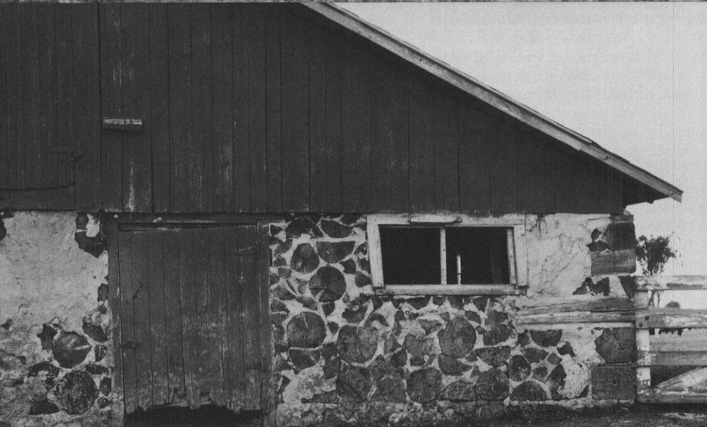
These three barns are typical of the massive stovewood construction found west of Green Bay. The stovewood section of the Rosera barn ( top ) was added around 1909 and is a good example of werkgerecht . The Wilcox barn ( center ) features exceptionally long quoins and mixes stovewood and fieldstone masonry. Of modified saltbox profile, the Mastey barn ( bottom ) is exceptionally massive.
