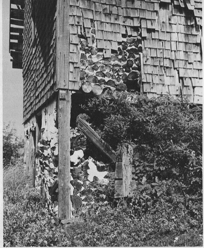
Also on the Zachow property are the remains of a stovewood granary. Exterior stovewood walls were generally shingled, clapboarded, or covered with vertical boards.
