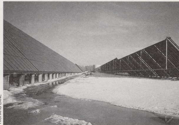
Packerland Packing Co. in Green Bay, the world's largest use of flat-plate solar collectors to produce hot water.
