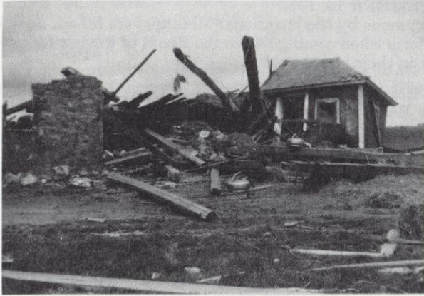
Tornado damage at Albert Podevel farm.
