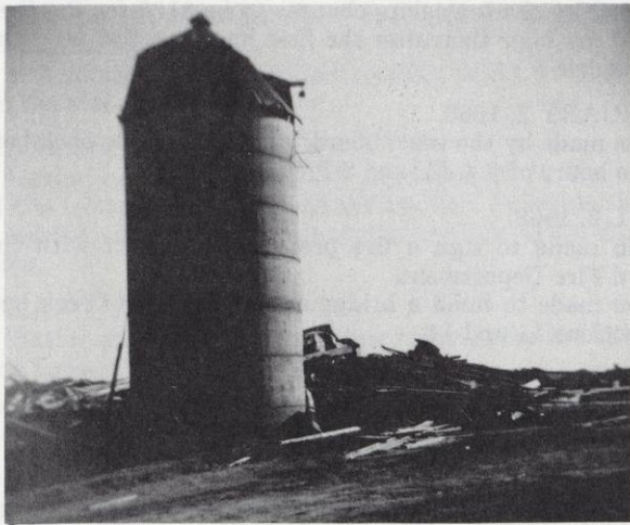
Tornado damage at Elmer Mueller farm.
