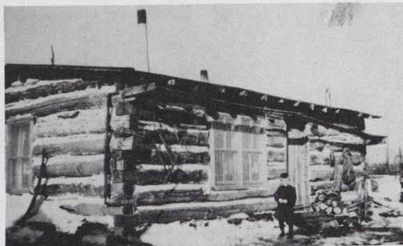
Log house owned by Prof. Williams on Bendel Fram before Bender owned it.
