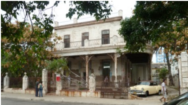
Figure 31. Exterior of building on Calle Línea #504, e/D y E, Vedado, Havana, Cuba. Site of Crispin Gurholt, Live Photo #23: Havana, Cuba , 2012, installation and performance, photo by author
