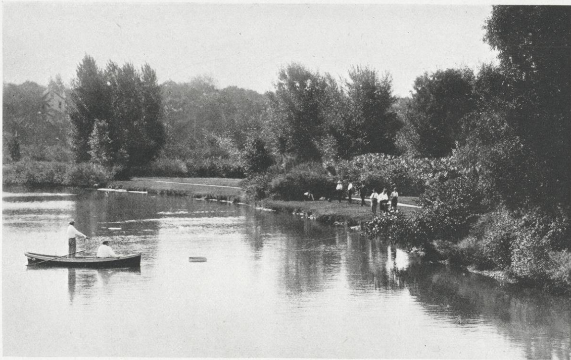
CASTING, TENNEY PARK LAGOON
