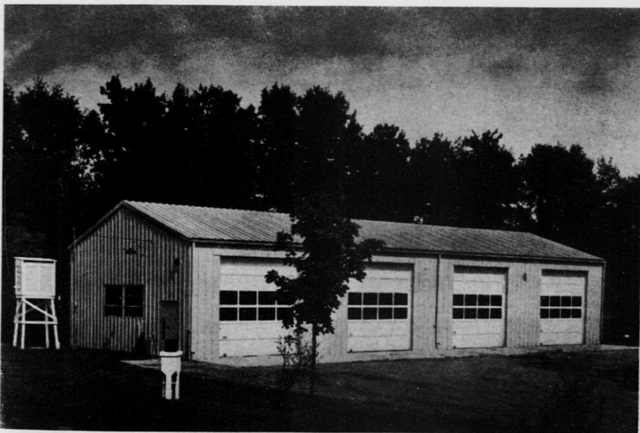
Once government surplus, this steel building now provides needed shop and storage space at Wautoma.
