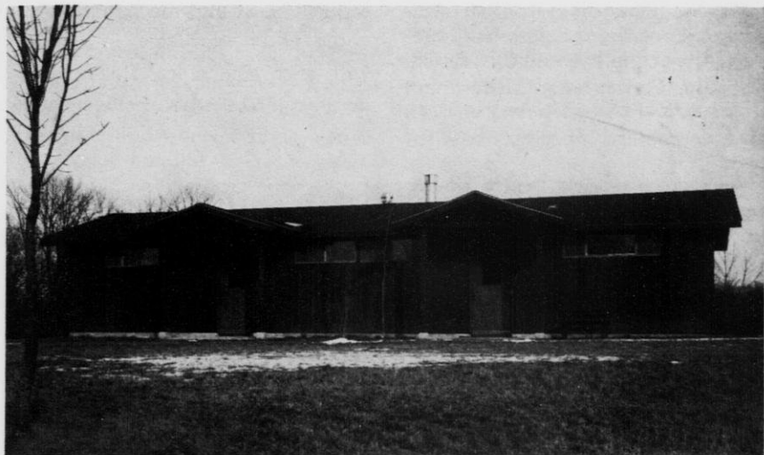
This is a new youth camp dormitory at Wyalusing state park.
