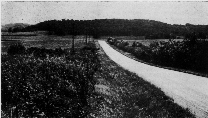
Low-growing brush is selectively managed along the left side of this road. The result is an attractive highway with food and cover for wildlife, but without the safety hazards of tall-growing brush.
