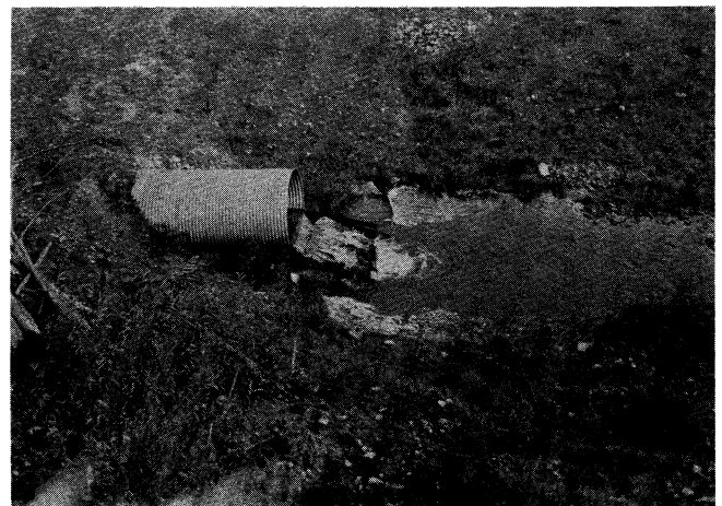
The fish barrier impounded a shallow pool upstream (left) and scoured out a 4½-foot splashpool downstream (right).
