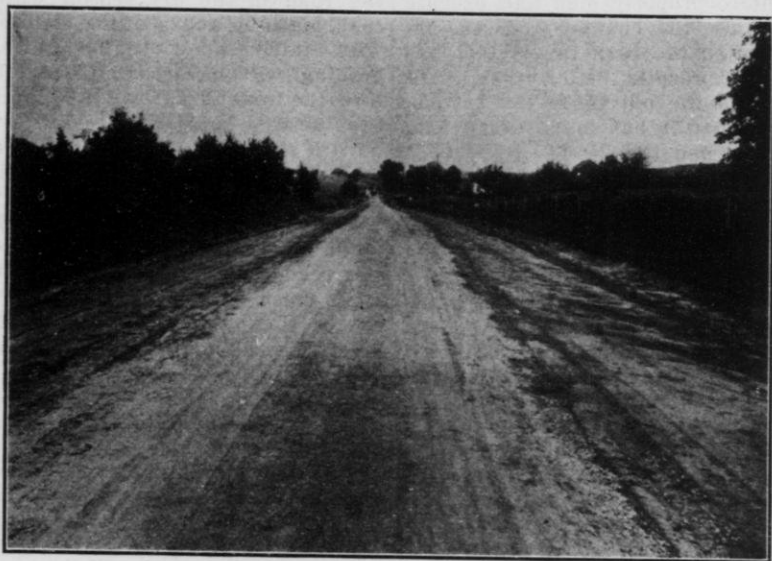
Whitewater and Fort Atkinson Road, Town of Koshkonong, Jefferson County. Crushed Limestone from quarry, 1913. R. D. Royce, County Highway Commissioner.
