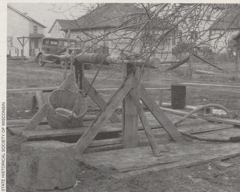
This open well served a Wood County family in 1934. Surface runoff flowed into unsealed wells, contaminating groundwater with bacteria. To protect public health and groundwater, the 1936 Wisconsin Well Code set standards for proper well construction.
