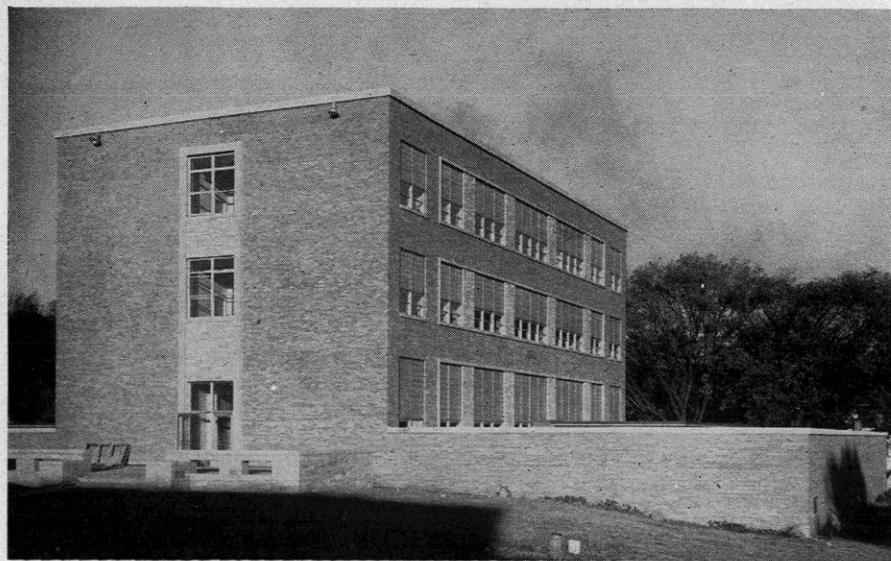
HERE IS WISCONSIN'S center of chemical engineering education and research, the University of Wisconsin's new Chemical Engineering Building, which has gradually been put into full use on the UW campus during this semester as installation of its technical equipment is completed in its 10 laboratories. The building, completed at a cost of $885,000, is located on the Engineering campus off Randall Avenue. Of the construction funds, $500,000 came from the Wisconsin Alumni Research Foundation (WARF) and $385,000 from state appropriations. The building has three stories and basement constructed of concrete, lannon stone, and brick, and besides the 10 laboratories, it provides classrooms and offices and other special service and work rooms for the University's chemical engineering staff and students.
