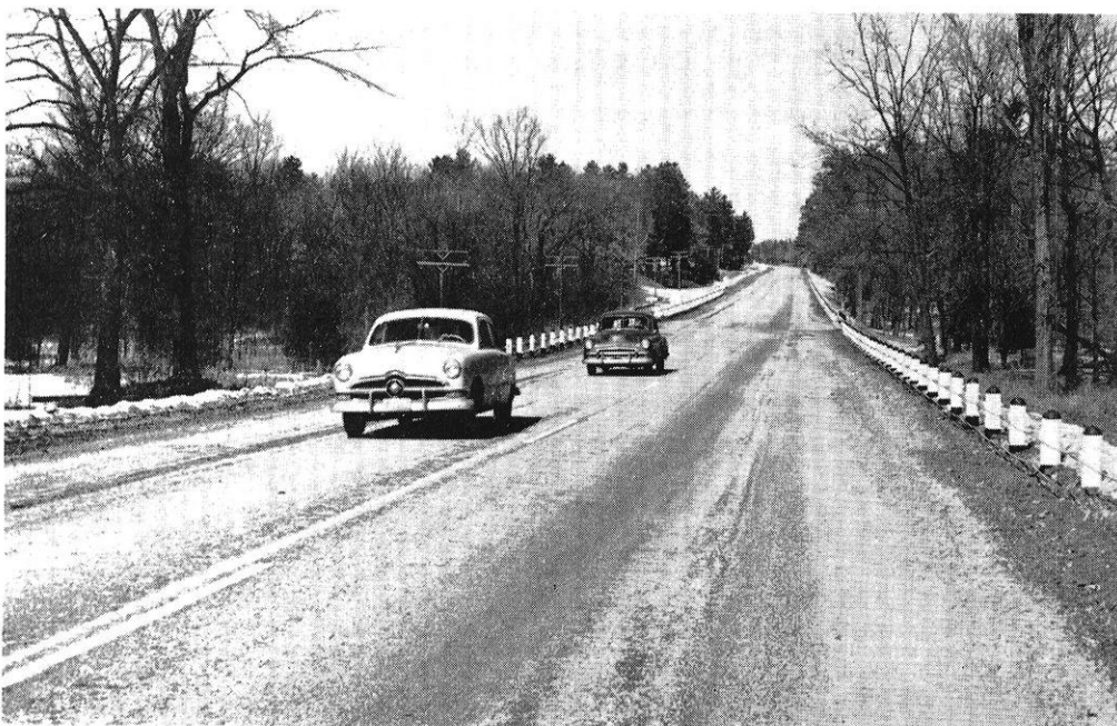
Fig. 1.—This soil-cement road, Route 13 in Adams County, Wis., was one of the first built in the Midwest. It is still giving good service after nearly 20 years of use. Samples of the pavement taken in 1954 tested 2,800 psi compressive strength, nearly five times the 640 psi strength of 7-day specimens taken when the road was built.
