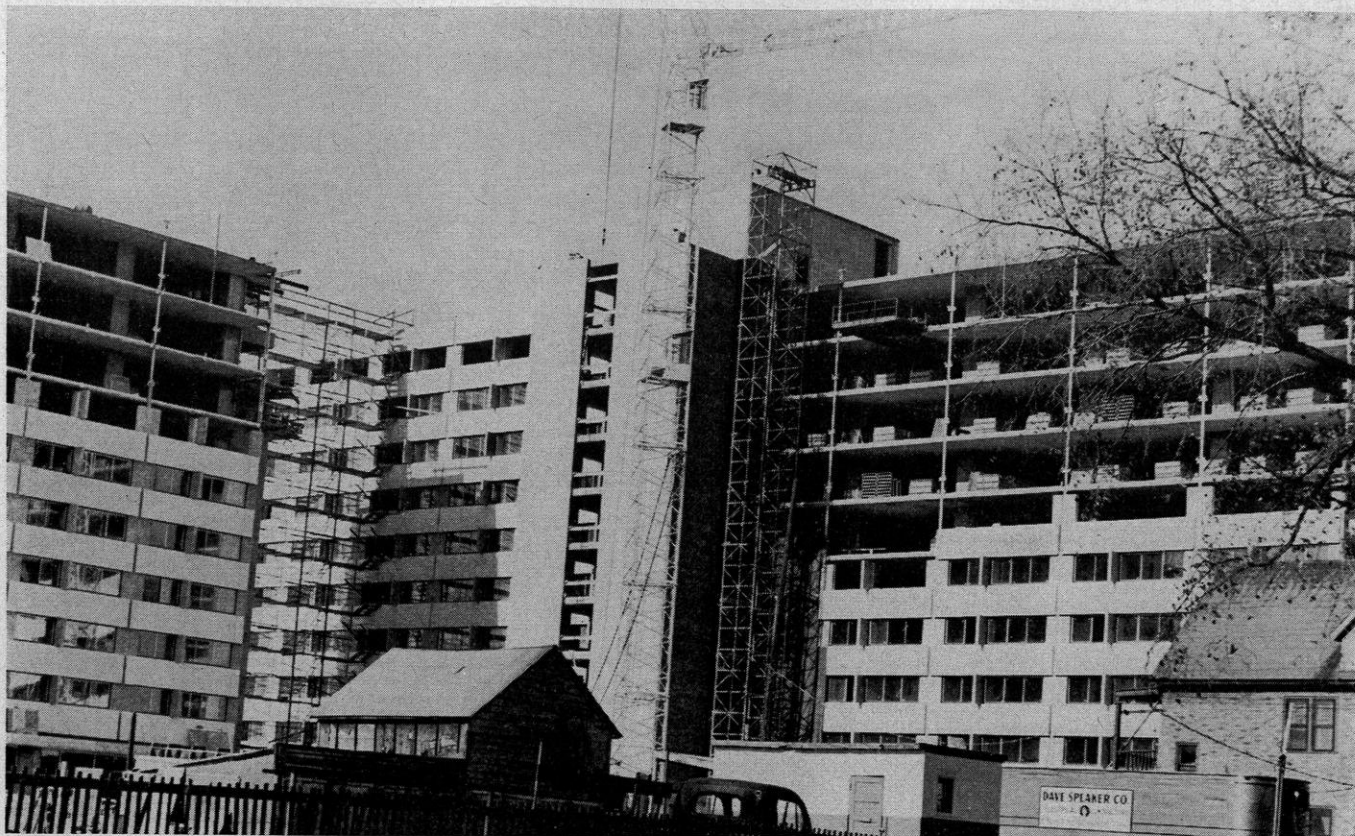
Witte Hall—Southeast Dormitories
