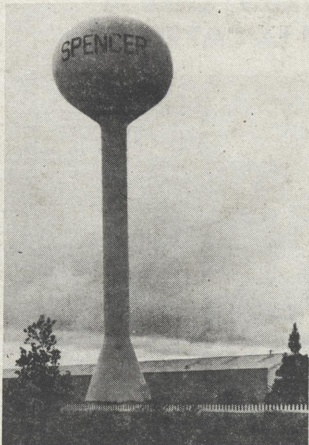
SPENCER WATER STORAGE FACILITY — The population of Spencer enjoys a quality of water service provided by much larger cities. Significant improvement in the system was made in 1966 when an additional storage tank of 200,000 gallon capacity, (pictured above) was put into service. A tank constructed in earlier years, still in use, has a capacity of 50,000 gallons. Spencer's good water, with top pressure for fire protection, is derived from a system of three wells. (News-Herald Photo)
