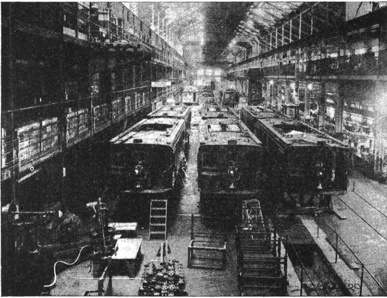
In these shops have been built the electric locomotives for railway electrifications in America as well as numerous other countries.
