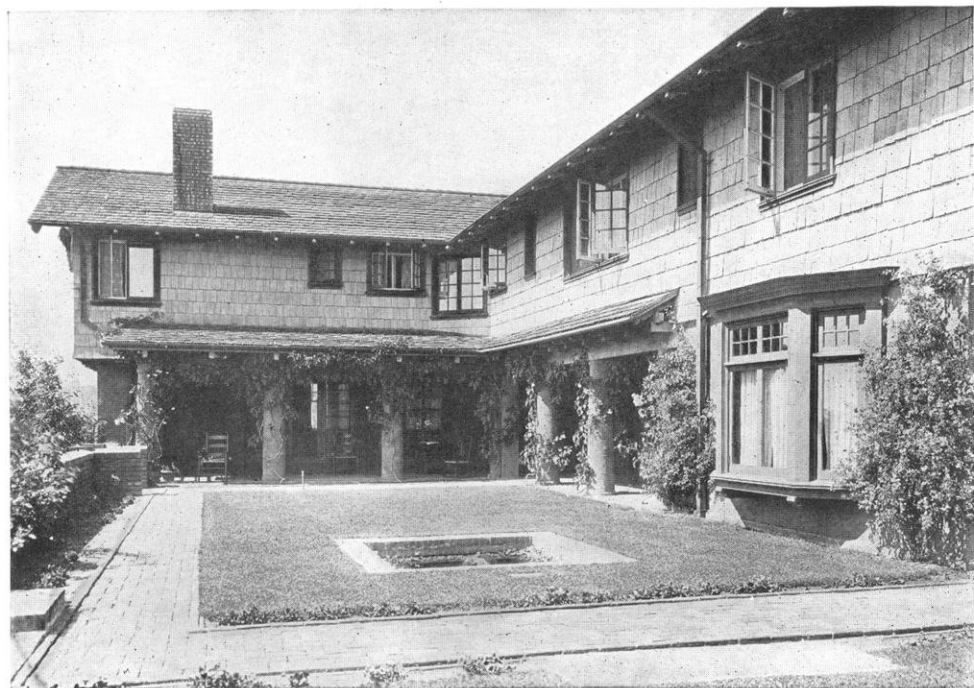
FRONT VIEW OF TOWN HOUSE BUILT AT SANTA MONICA, CAL., BY MESSRS. MYRON HUNT AND ELMER GREY.
