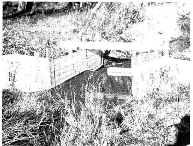
Two-step weir used in gaging flow of Pheasant Branch South.
