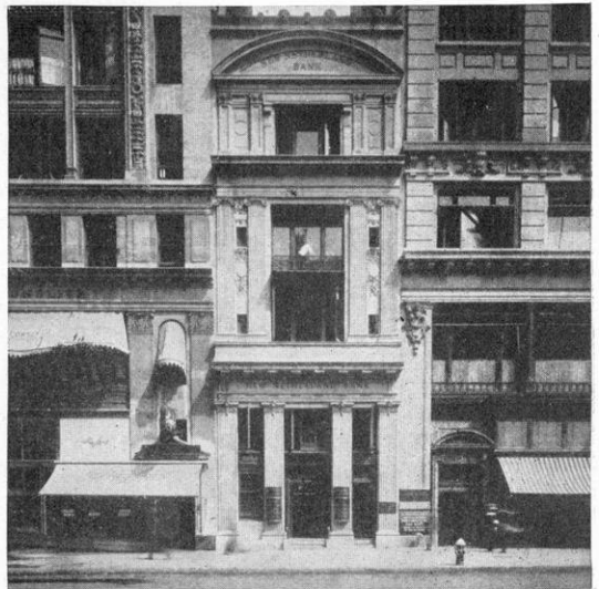
THE BUILDING OCCUPIED BY THE CRAFTSMAN MAGAZINE, AT 41 WEST 34TH STREET, NEW YORK.
