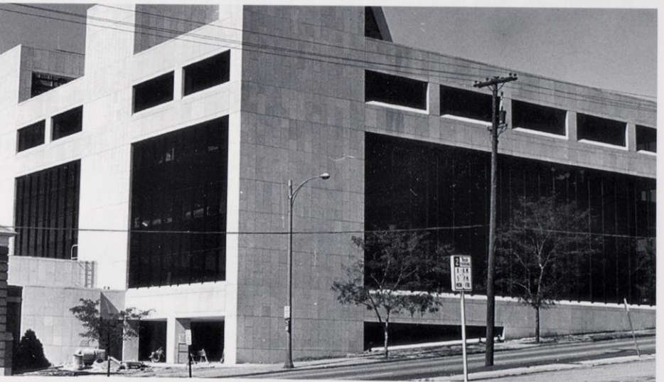
In September 1981, Parker Pen completed renovation and expansion of its worldwide headquarters at South Parker Drive and East Court Street in downtown Janesville. The building was re-covered with a new exterior consisting of 336 travertine panels, each weighing more than a ton. The photos above show the project's progress from the building's original brick exterior to partial re-covering and finally to the new exterior. After the headquarters moved to Europe, the building was later bought and renamed for its address, One Parker Place.
