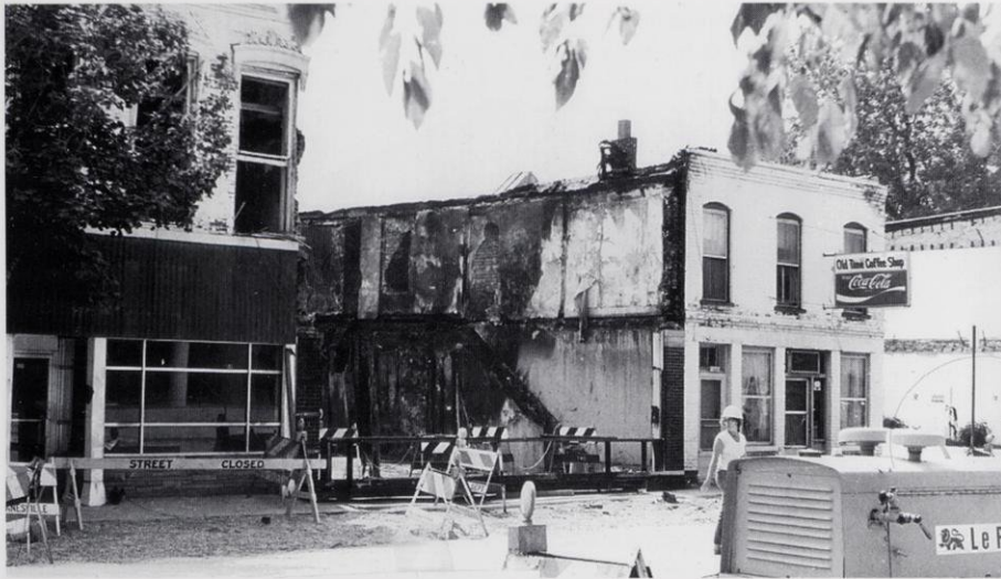
A natural gas explosion and fire leveled the Agnew & Porter Law Office at 107 N. Main on June 1, 1981. More than a dozen people were injured when city workers ruptured a gas line while digging a trench for a new sewer. The buildings on both sides of the explosion were razed.
