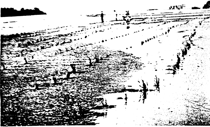
Figure 2. Photograph showing placement of smooth cordgrass plugs on 1 m centers with rows 2 m apart..
