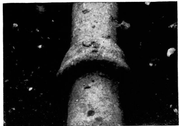
This 123-year-old cast iron water main is still in use in the distribution system of St. Louis, Mo.
