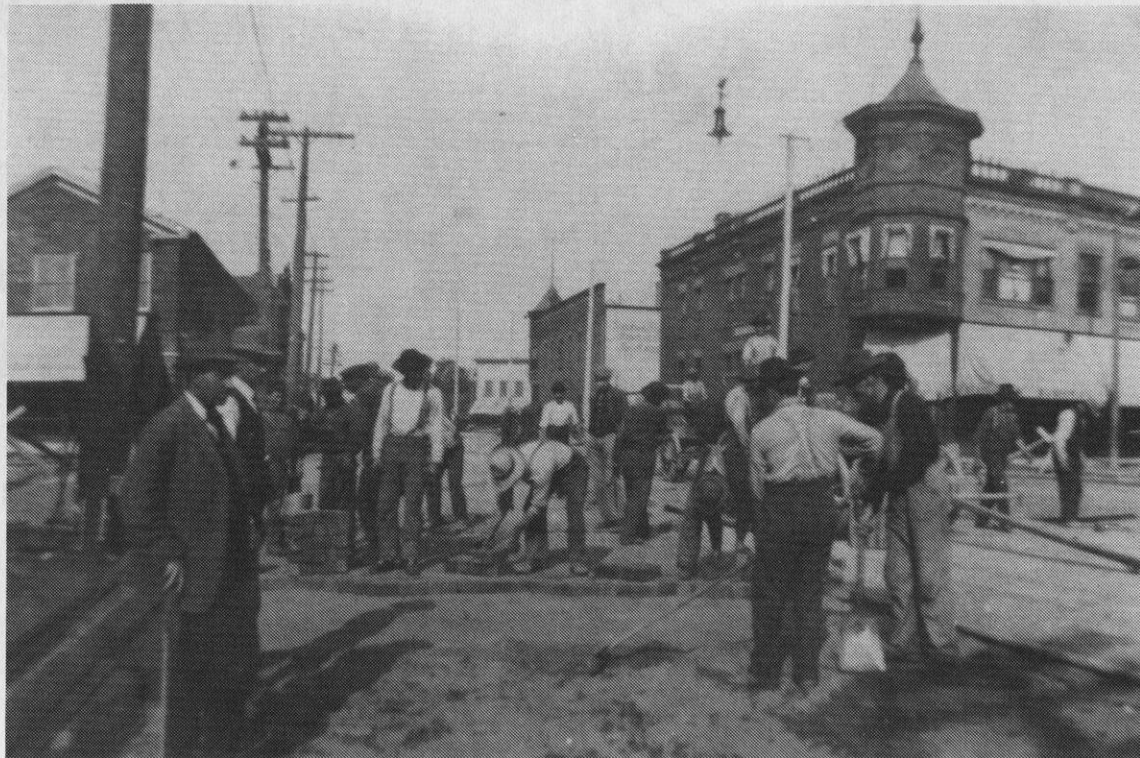
LAYING TRACK & STREET BRICK CORNER OF GENEVA & CHESTNUT 09
