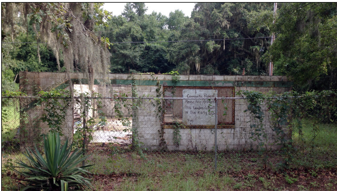
Figure 5 The Progressive Club, seen from River Rd. in August 2014. Photo by author.
