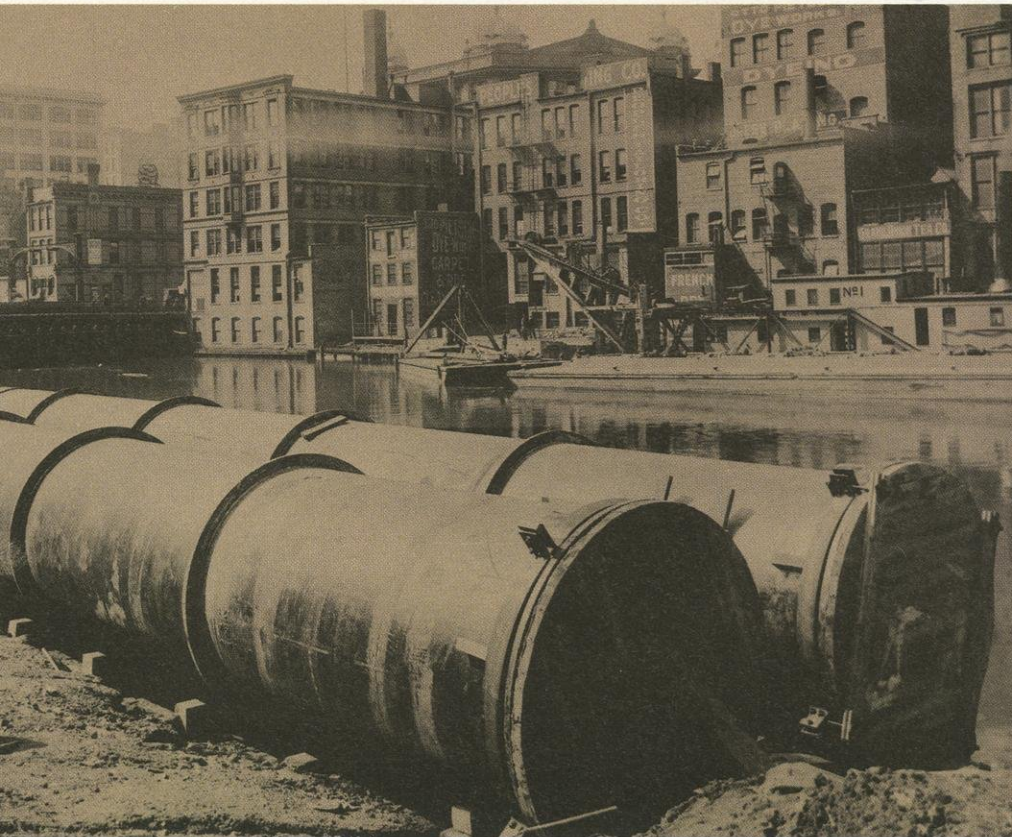
WISCONSIN ELECTRIC POWER CO.
