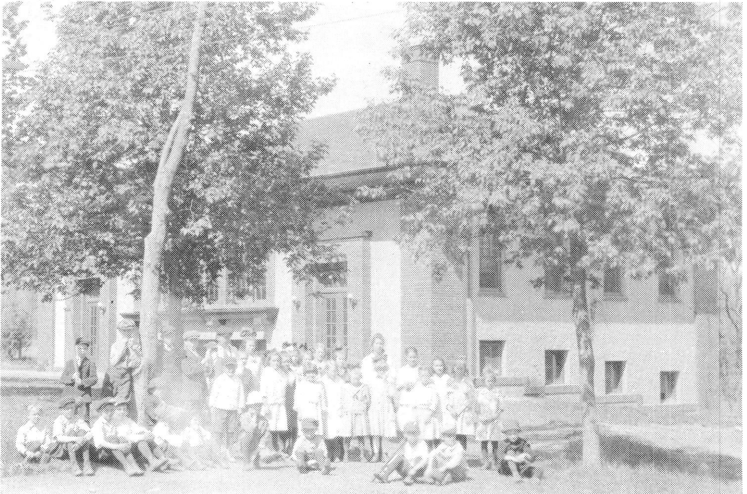
District 6 "Nakoma" School completed in 1917. After the additions were put on, the entry doors as shown here were removed. Children not identified. (Courtesy, Stark Company)
