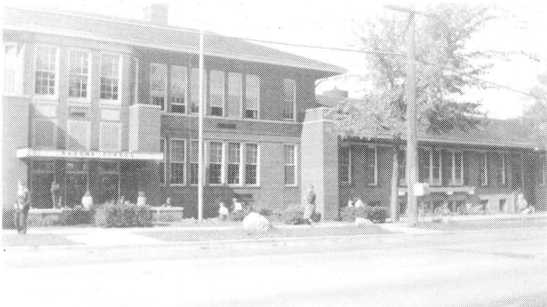
Nakoma School. The portion of the building behind the mailbox was the original building built in 1917. The eastern addition is partly seen on the right side of the photo. The two story portion of the building was the addition built in 1928.
