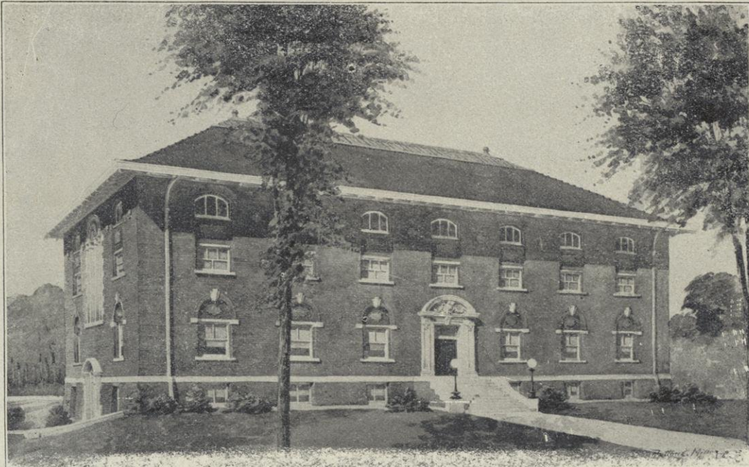
NEW GYMNASIUM—BELOIT COLLEGE.
