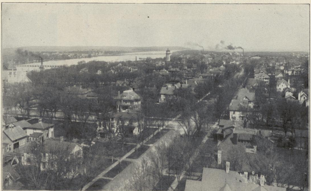
BIRD'S-EYE VIEW OF CHURCH STREET.
