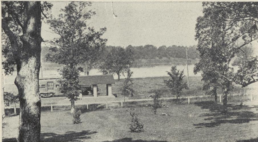
View from Clubhouse Across River, Country Club Interurban Station.
