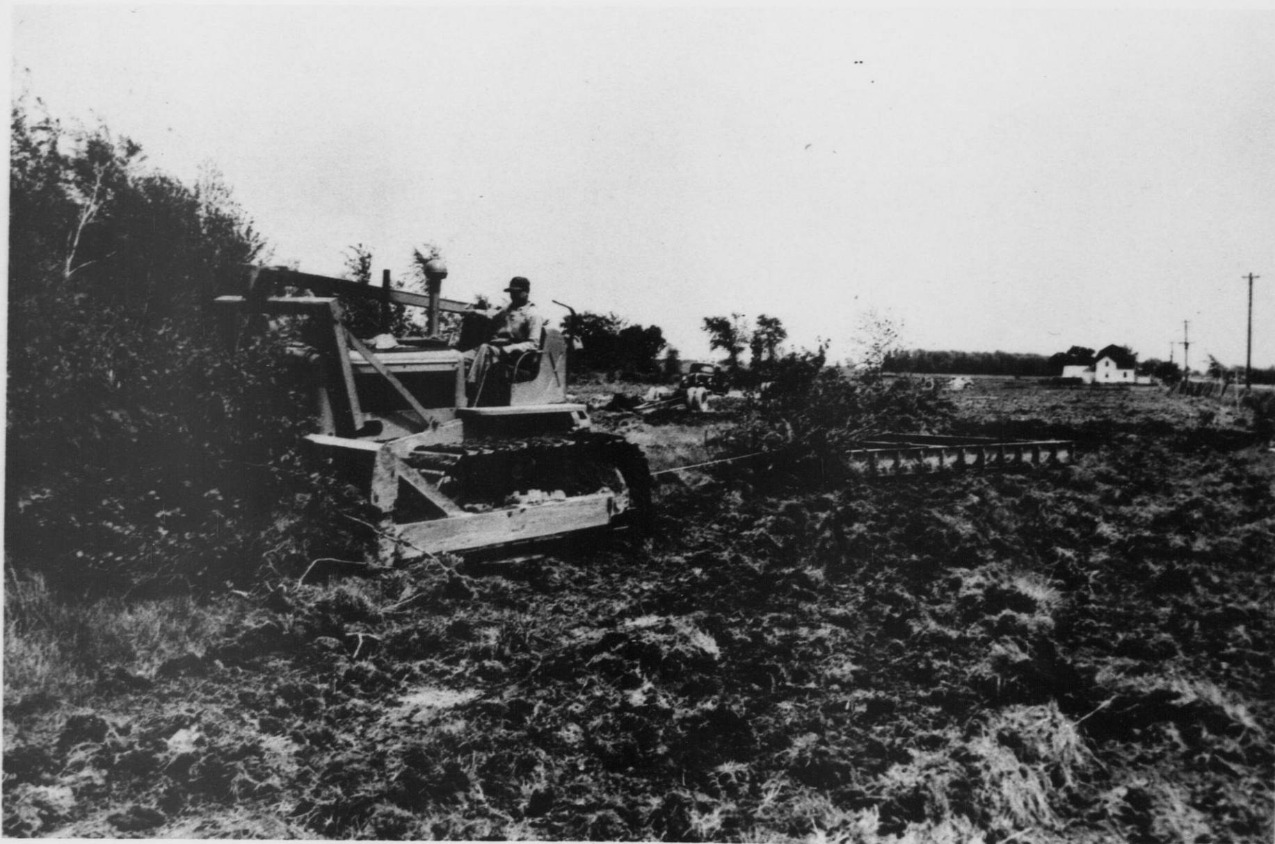
One phase of soil conservation is good land use. The two-ton steel A-Drag owned and operated by the Soil Conservation District leveled or cleared about 500 acres of stumpy land in 1949 to be used for pasture, thereby helping to lighten the crop load on present crop land.
