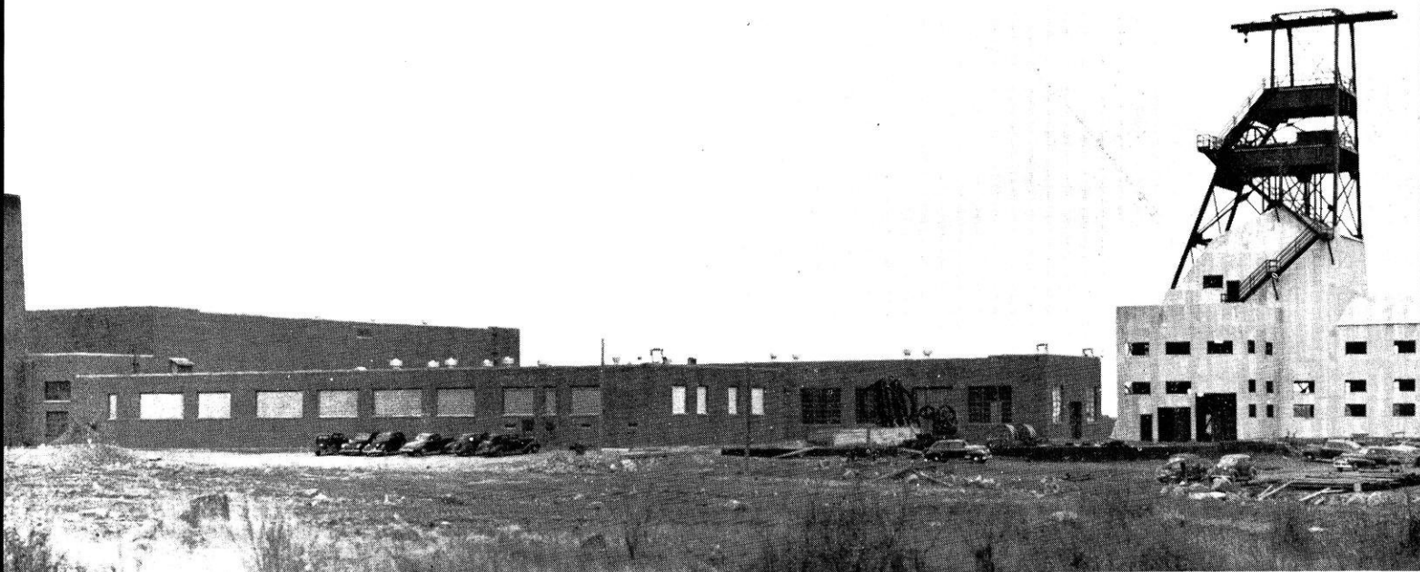
A general view of the Cary Mine surface plant.
