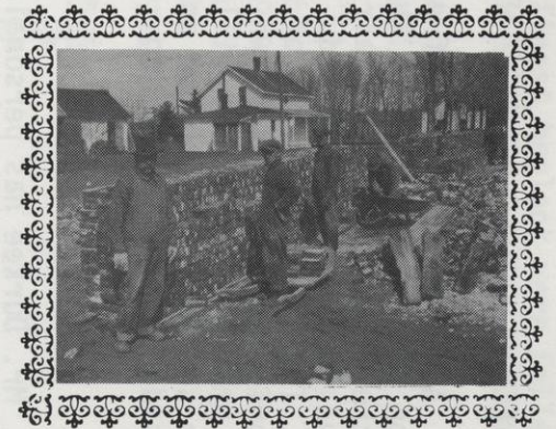
NEARLY ALL THE DEBRIS HAS BEEN CLEANED UP.
