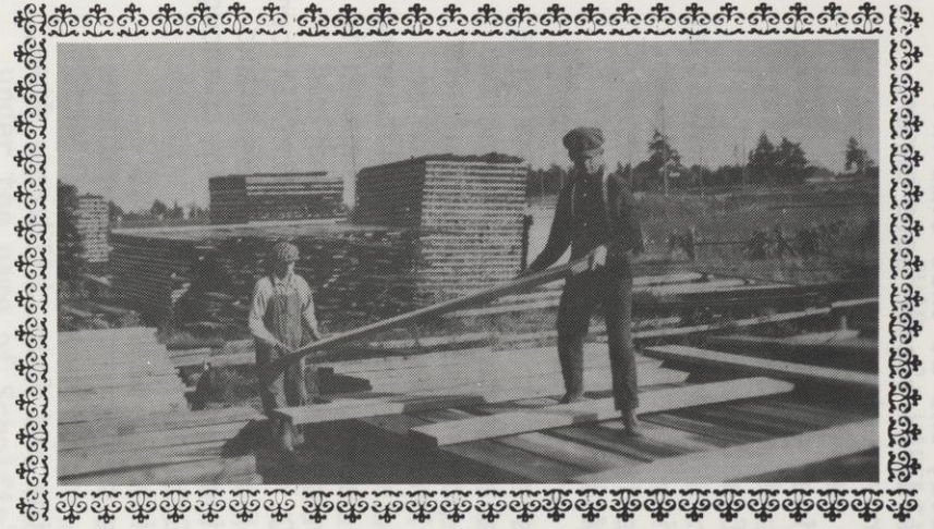
ANOTHER PILE IS BEGUN
