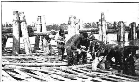
Weaving mattress for dike on Missouri River. Note pile bent in background.
