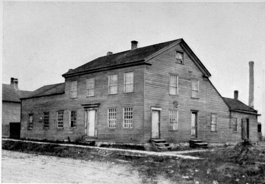
First Frame Building Erected.
