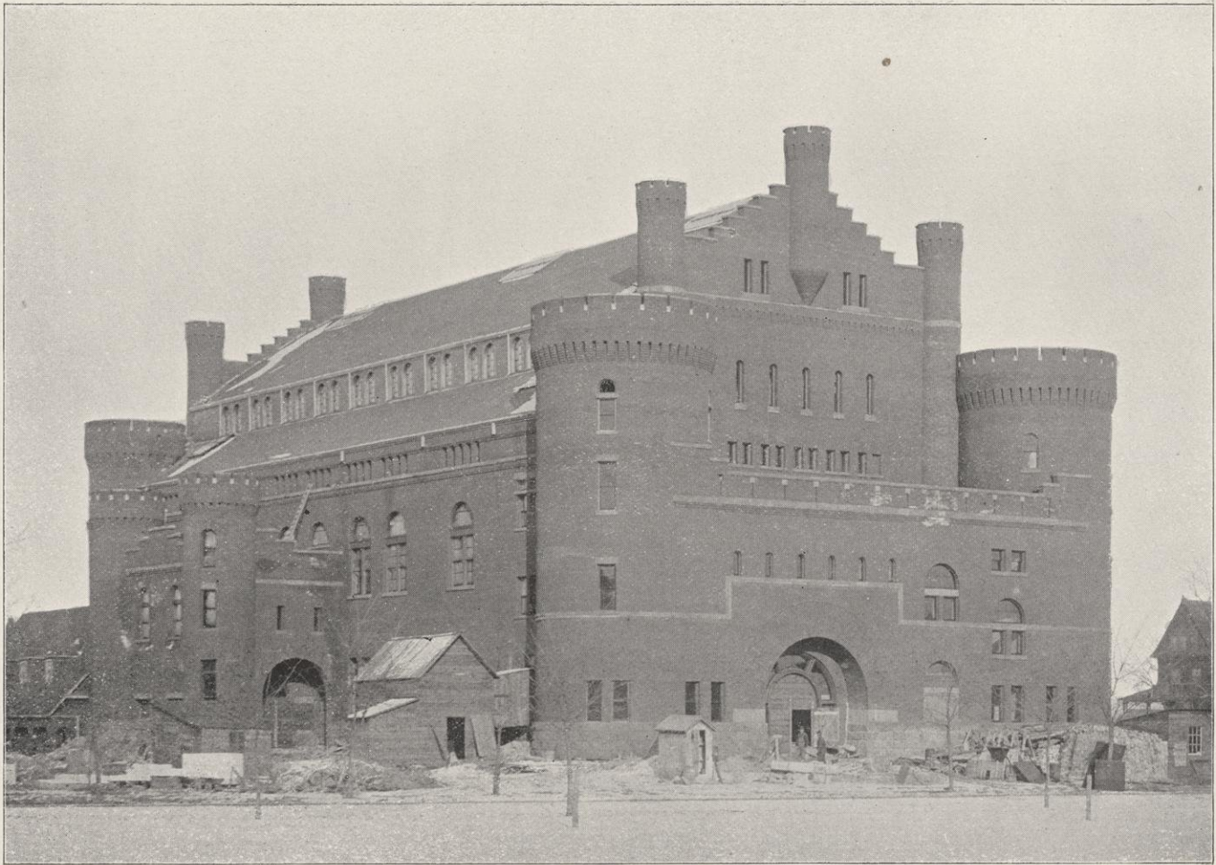
GYMNASIUM IN PROCESS OF CONSTRUCTION.
