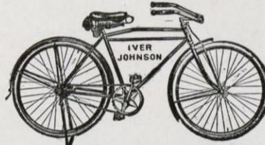
Iver Johnson is the only Bicycle built today of high Carbon "SEAMLESS" steel tubing.
