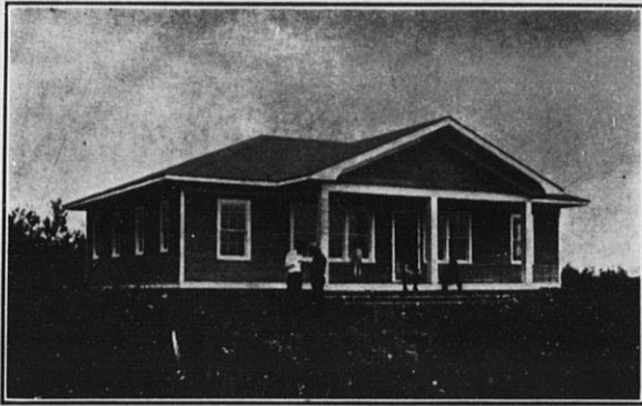
Community Building at Meadowbrook
