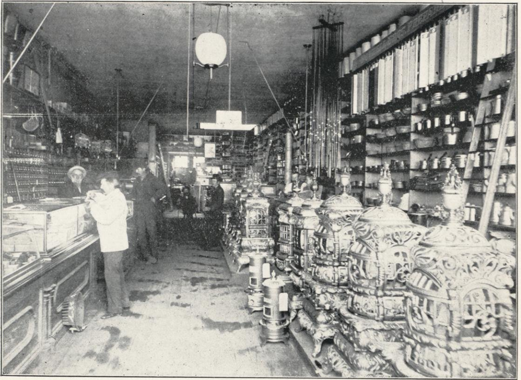
INTERIOR VIEW C. A. DEWEY'S HARDWARE STORE.
