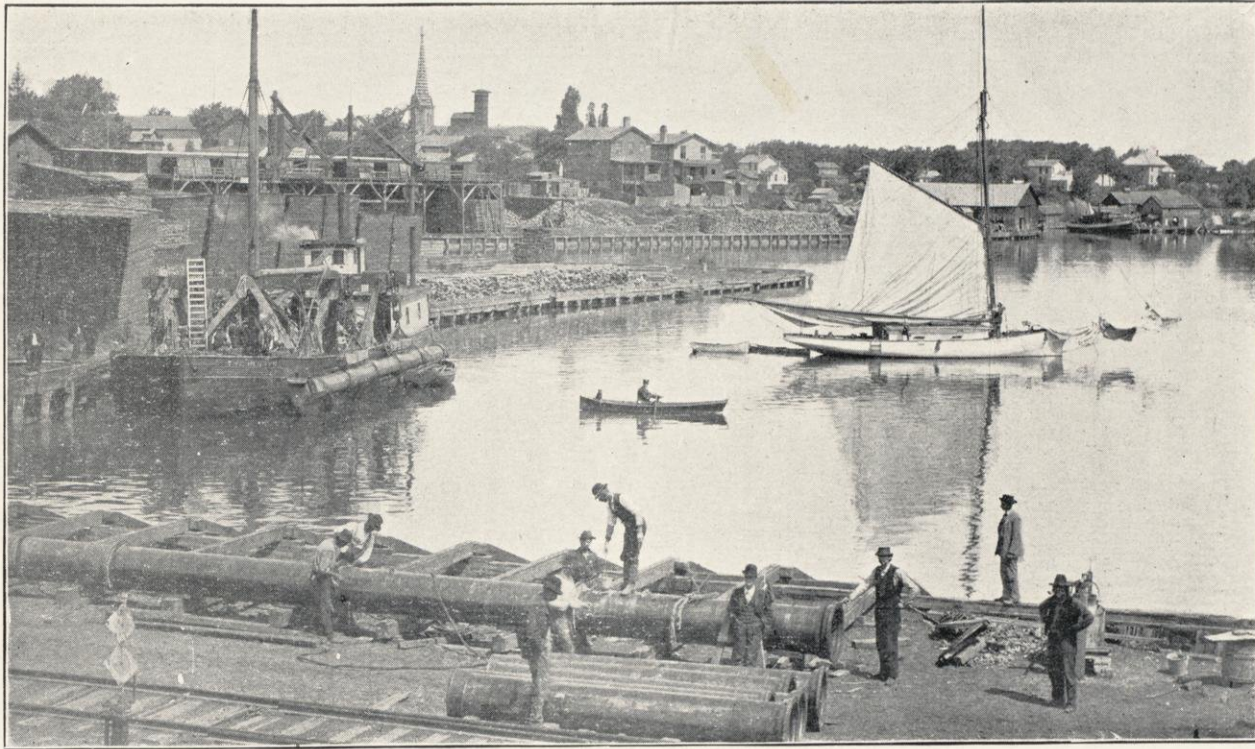
KENOSHA HARBOR—PREPARING INTAKE PIPE FOR CRIB.
