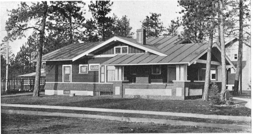
A BUNGALOW IN SPOKANE, WASHINGTON, COVERED WITH RUBEROID ROOFING, WHICH IS ESPECIALLY IN KEEPING WITH THE LONG, LOW LINES OF THE BUILDING: THE PHOTOGRAPH IS REPRODUCED BY PERMISSION OF THE STANDARD PAINT CO.
