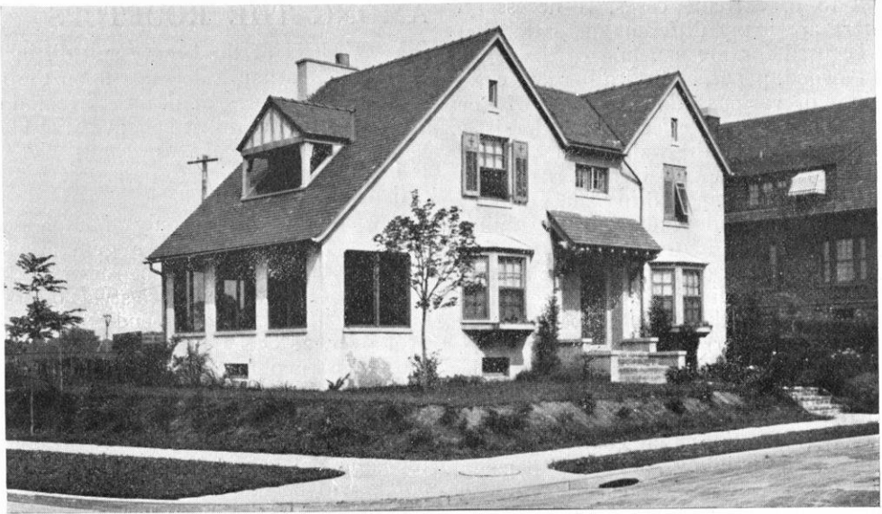
THE ROOF OF THIS INTERESTING LONG ISLAND HOUSE IS COVERED WITH TRANSITE ASBESTOS SHINGLES MADE BY THE H. W. JOHNS-MANVILLE CO.
