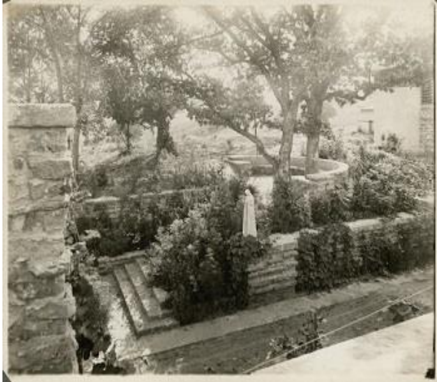
Figure 26. Wright embraced a rugged naturalism on the grounds of Taliesin I as seen in a summer view of the Tea Circle. His sculpture, Flower in the Crannied Wall , was placed in a prominent position facing the residential wing. (Courtesy the Wisconsin Historical Society, Henry Fuermann and Sons, ca. 1911).
