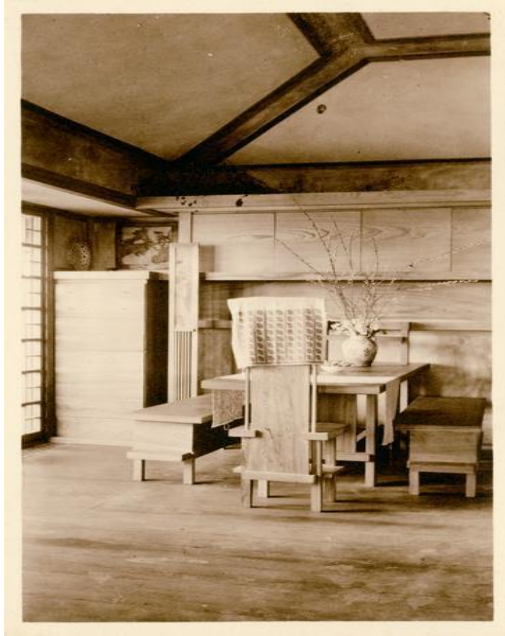
Figure 29. Taliesin I dining area displaying Wright’s use of wood and paint as ceiling decoration which emphasized the verticality of the space (Courtesy the Wisconsin Historical Society, Taylor Woolley, ca. 1911).
