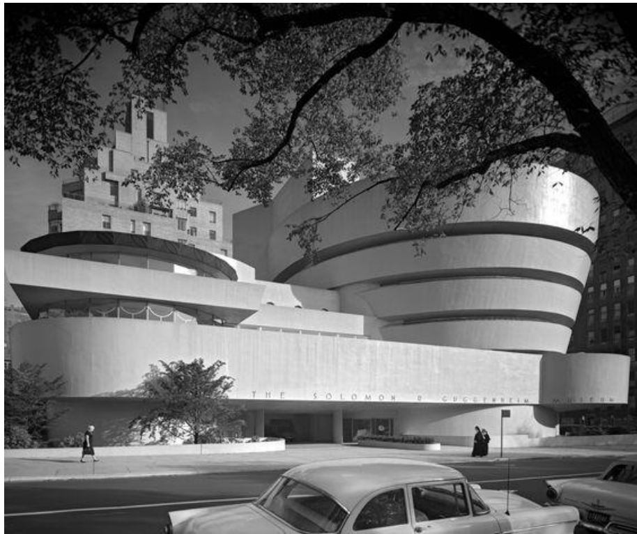
Figure 55. Wright's design for the Guggenheim Museum involved two primary forms. The main gallery was conceived as a massive spiral form while the Monitor Building, to the left, was a far less dominant rotunda. A strong horizontal band connected the two elements and provided a covered space for the main entry and vehicular access (Courtesy the Solomon R. Guggenheim Museum Archives, Robert E. Mates, 1959).
