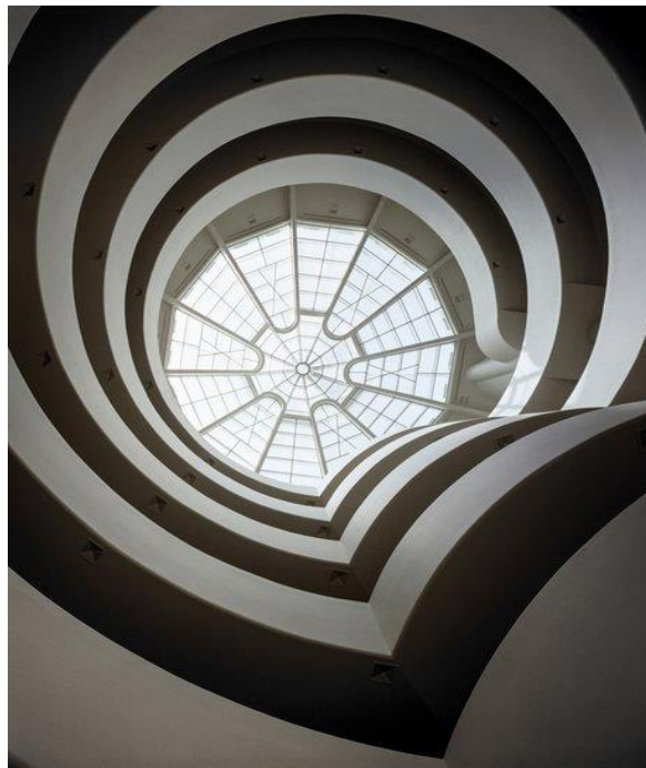
Figure 64. Wright created variation in the rotunda interior by intersecting the main spiral with a smaller spiral that created a contrasting ‘bump,’ as in the overlapping of a Venn diagram (Courtesy the Frank Lloyd Wright Building Conservancy, 2018).
