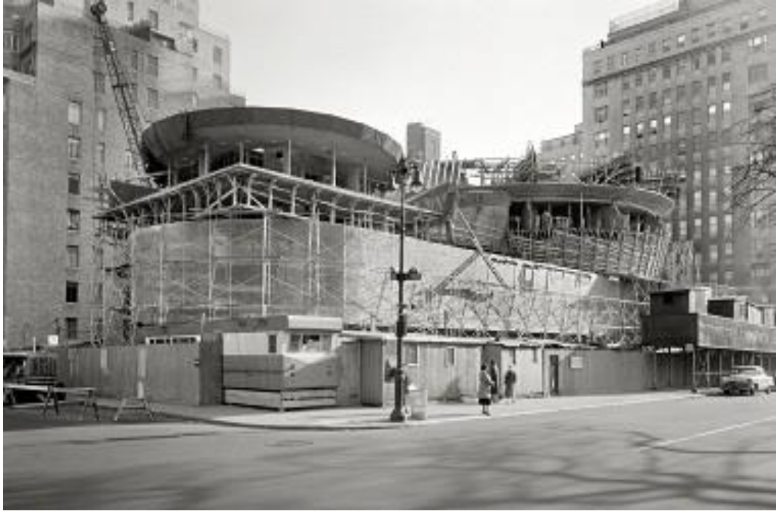
Figure 75. The final cost of the Guggenheim would be significantly higher than Wright's ongoing estimates as it was an enormously labor-intensive design. Construction of the shell involved the use of hand-built forms sprayed with liquid concrete called Gunitite (Courtesy the Solomon R. Guggenheim Foundation, Gottschleisner, 1957).
