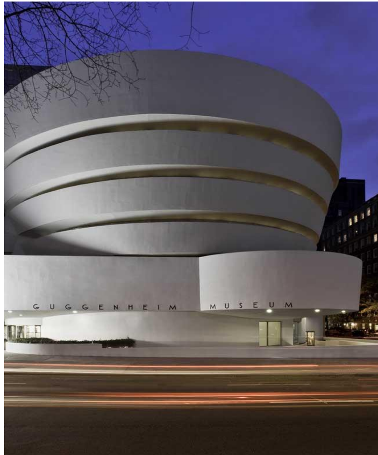
Figure 62. Wright made masterful use of cantilevers throughout his career as an architectural element of gravity-defying suspense. He incorporated a cantilever in the southwest corner of the Guggenheim Museum (Courtesy the Solomon R. Guggenheim Museum, Robert E, Mates, ca. 2000).
