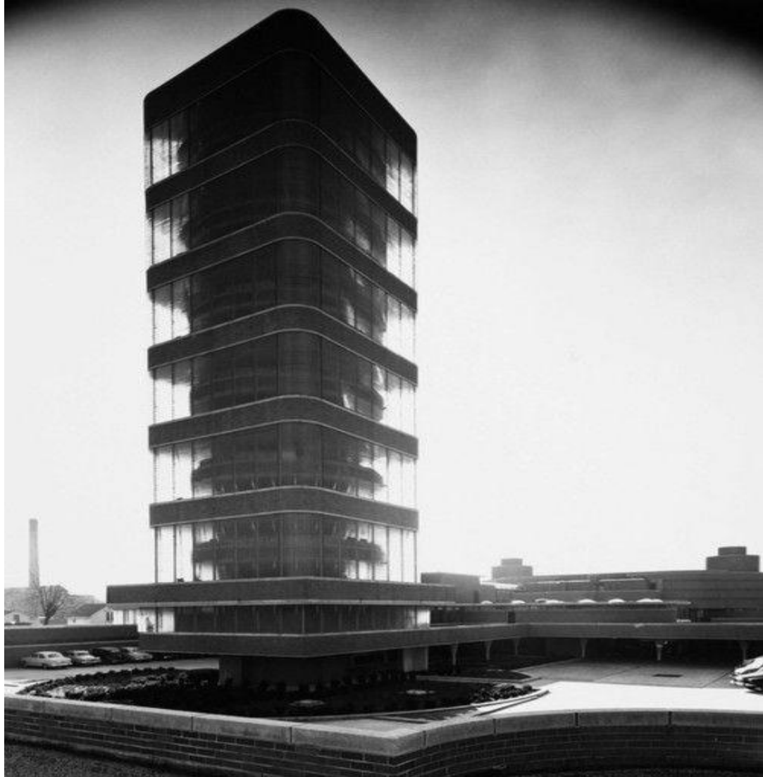
Figure 51. Johnson Wax Research Tower showing interior core from which floors and glass curtain walls were cantilevered (Courtesy SC Johnson, ca. 1962).
