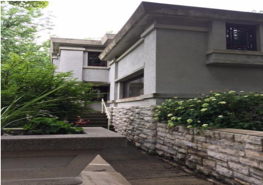
Figure 1. The Blythe House, designed by Walter Burley Griffin, is a prominent member of the Rock Crest/Rock Glen collection of Prairie School homes in Mason City, Iowa (Mark Dieter, 2018)
