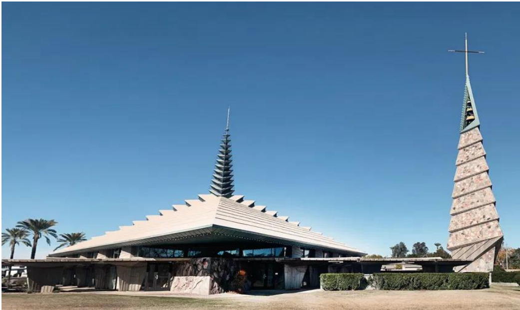
Figure 49. Wright's frequently incorporated spires in his architecture. This was the double-spire design for the Southwest Christian Seminary's chapel that was eventually built as First Christian Church, Phoenix, Arizona (ArchEyes, 2020).
