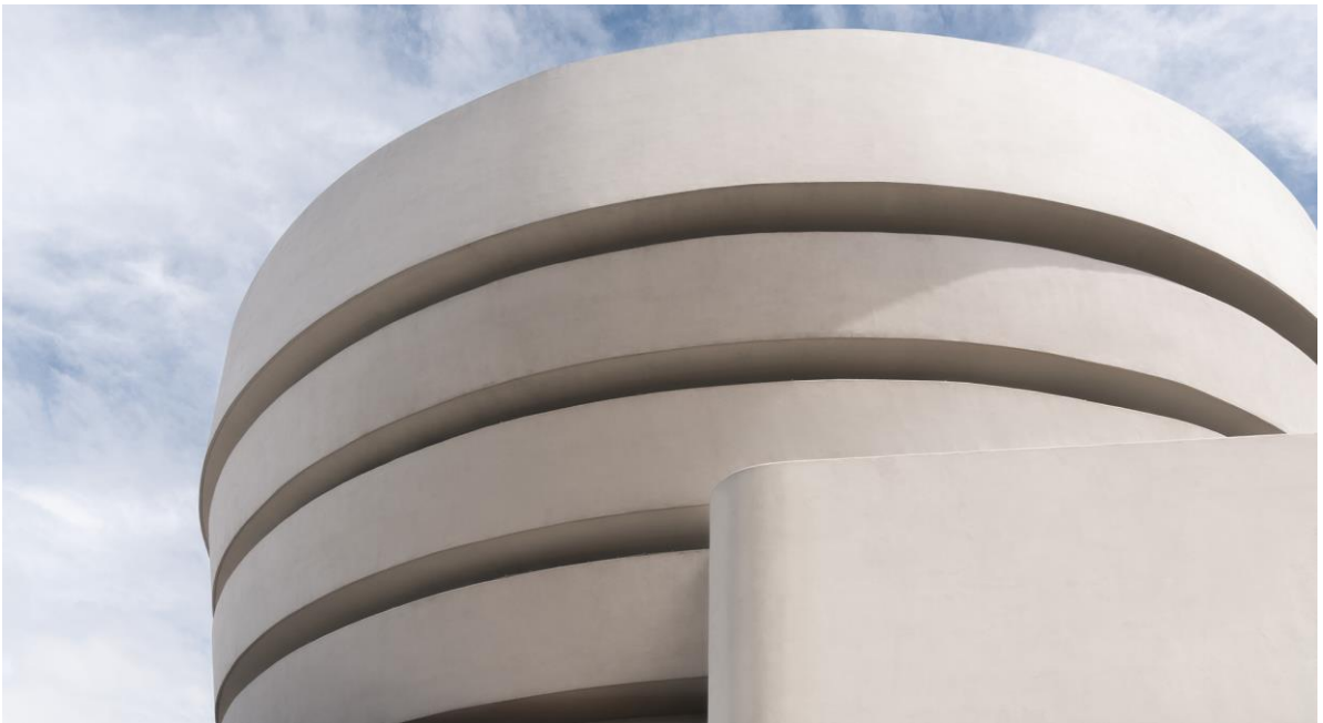
Figure 56. Wright accentuated the solid, exterior mass of the rotunda with deeply recessed striations (Courtesy the Solomon R. Guggenheim Museum, ca. 2000).
