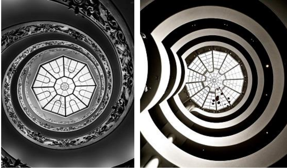
Figure 70. Guiseppe Momo designed an oculus (left) to provide dramatic effect with the Vatican staircase. Wright also incorporated an oculus (right) for natural lighting over the Guggenheim rotunda. (Dreamstime.com, Eliza Adamyan, 2015 and RobertoDeMicheli.com, Roberto DeMicheli 2012)
