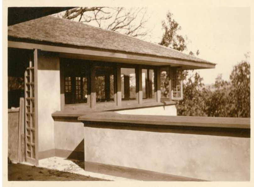
Figure 30. Wright designed an extraordinary number of windows for Taliesin I as seen in this image of the living room exterior. Numerous windows served not only to visually link the interior of the residence with the Valley but allowed seasonal fragrances to fill the home (Courtesy the Wisconsin Historical Society, Taylor Woolley, ca. 1911).
