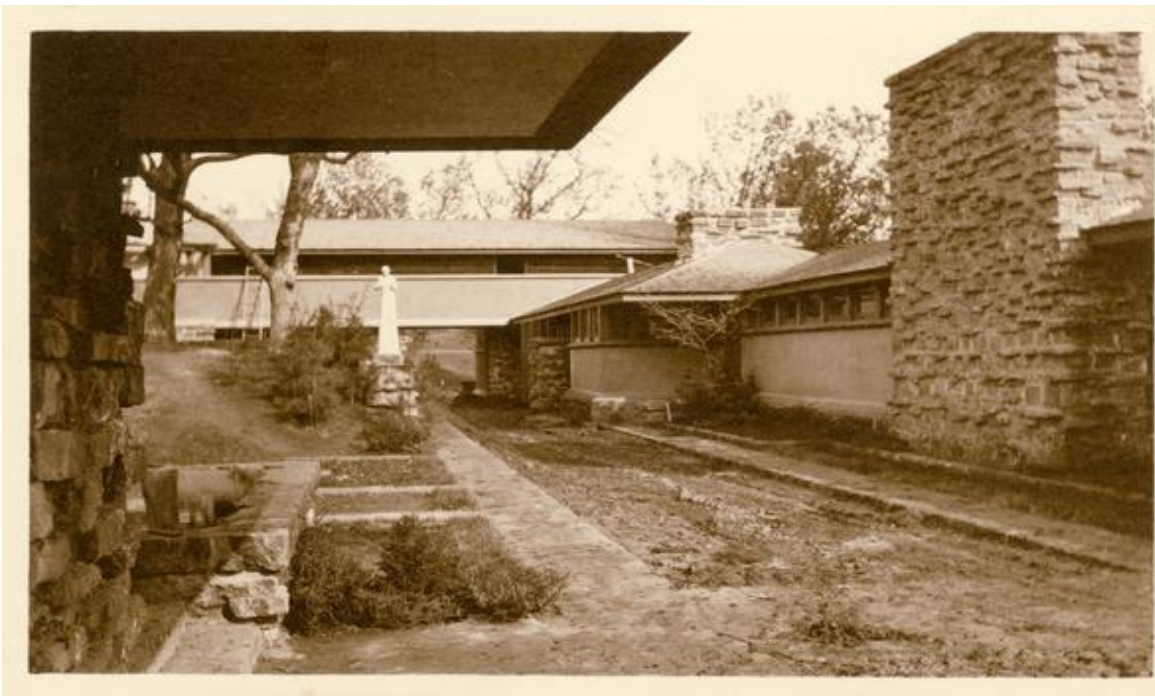
Figure 23. Wright incorporated a hayloft in the design for Taliesin I which looked like a covered bridge suspended on both ends. This was not only an important agriculture motif but framed the perimeter of the grounds (Courtesy the Wisconsin Historical Society, 1912).
