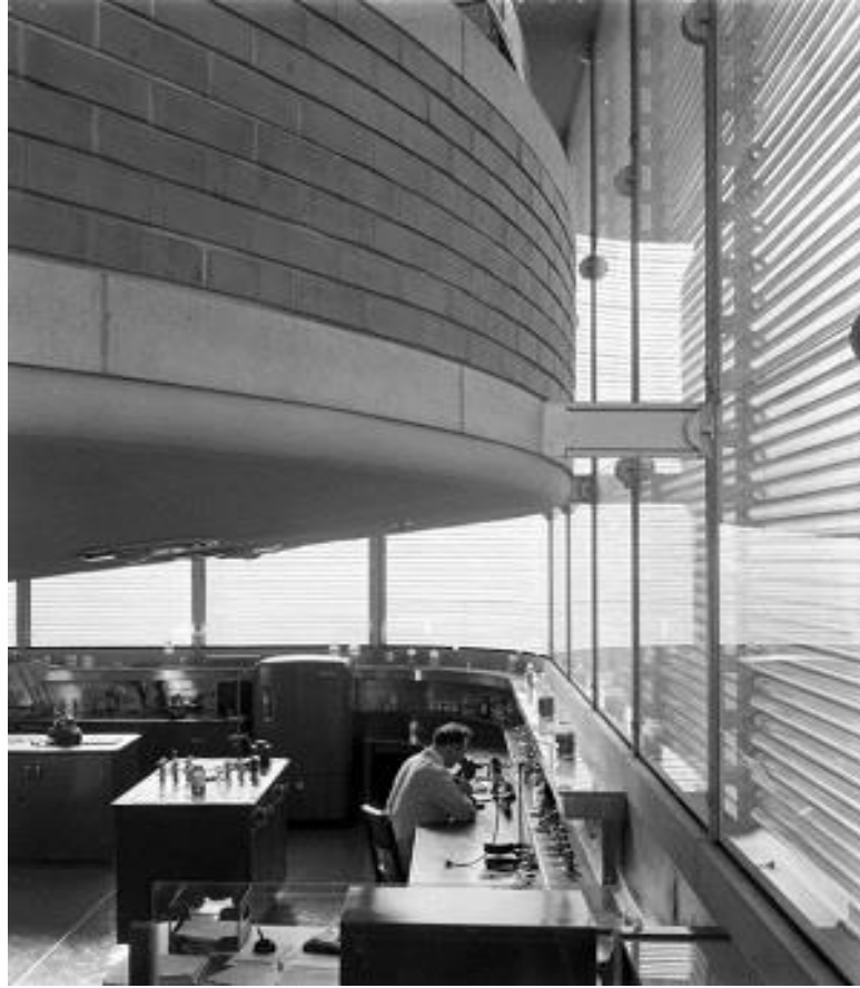
Figure 52. The radical design of the Research Tower with its use of glass walls and cantilevered floors provided both an inspiring and challenging environment in which to work (Courtesy SC Johnson, ca. 1955).
