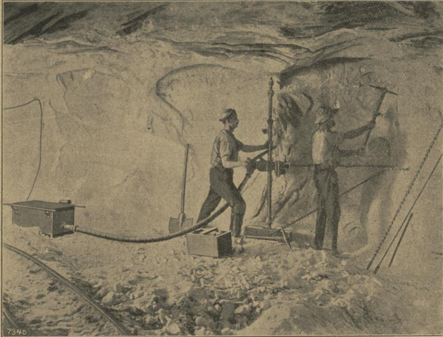
Electrical Drill in Operation.
