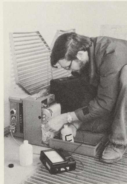
Ron Kazmierczak adjusts the strip chart on a recorder that keeps track of acidity from the plant at Manawa.
