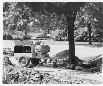
Le Roi portable air compressors are manufactured in 12 different models and used in the construction industry, in mining and quarrying, and by railroads and public utilities.
