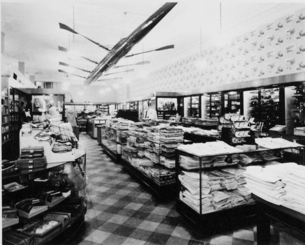
The C. W. Anderes Clothing Shop was one of several local businesses to lease space of the University Co-Op through the 1950s.
