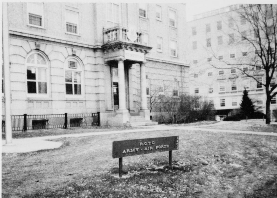
The Army and Air Force ROTC headquarters at 1402 University Avenue.
