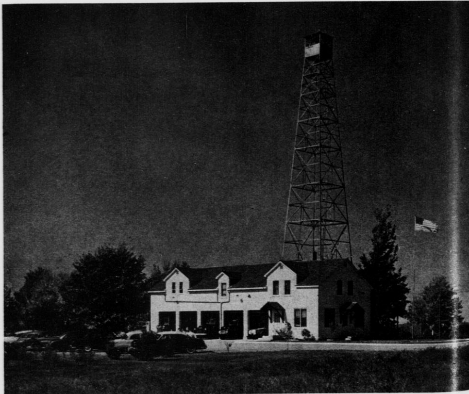
This is one of Wisconsin's subdistrict ranger stations.
